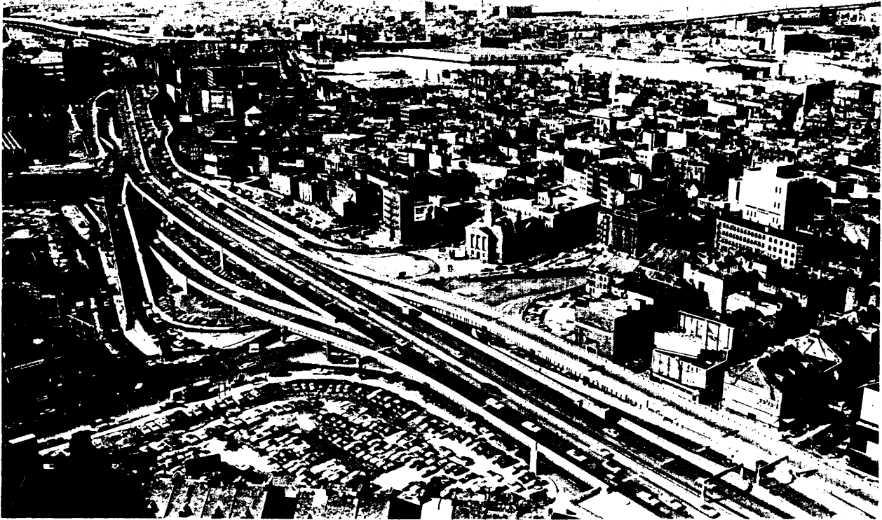
Highway construction issues dominated Boston's most significant recent transportation planning program, the Boston Transportation Planning Review
