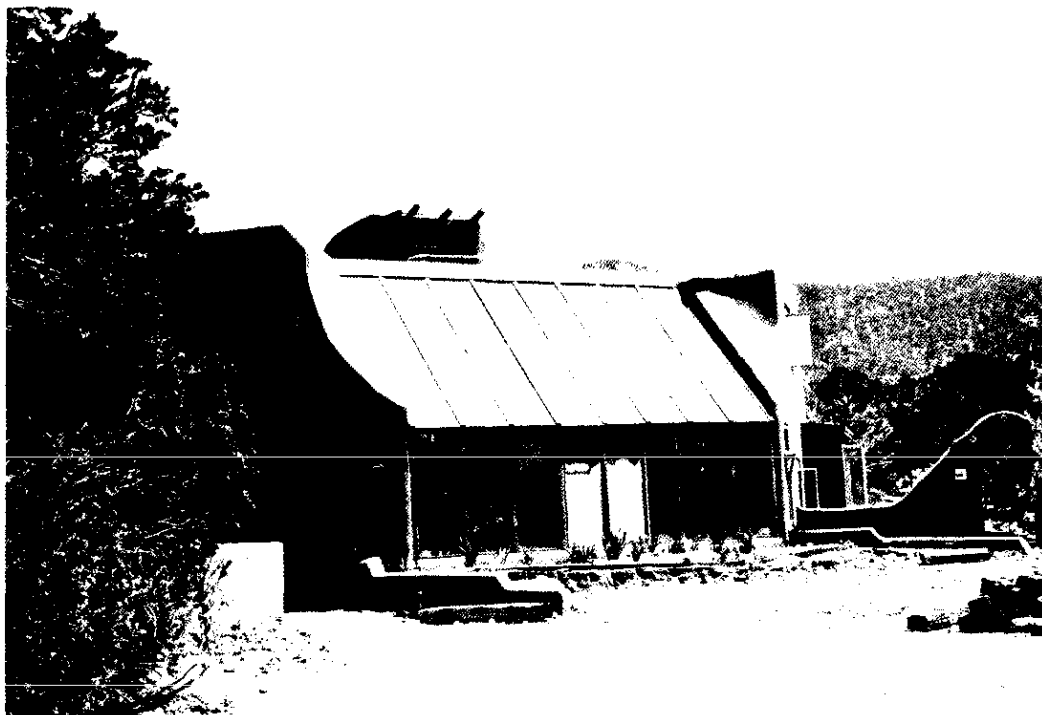
Figure 52.—The Balcomb Home Near Sante Fe, N. Mex., Combines the Use of a Greenhouse With a Rock Storage Bed to Provide 95 Percent of Its Heating Needs
