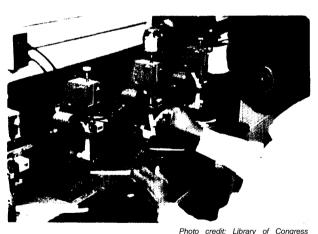
Fold endurance test apparatus
