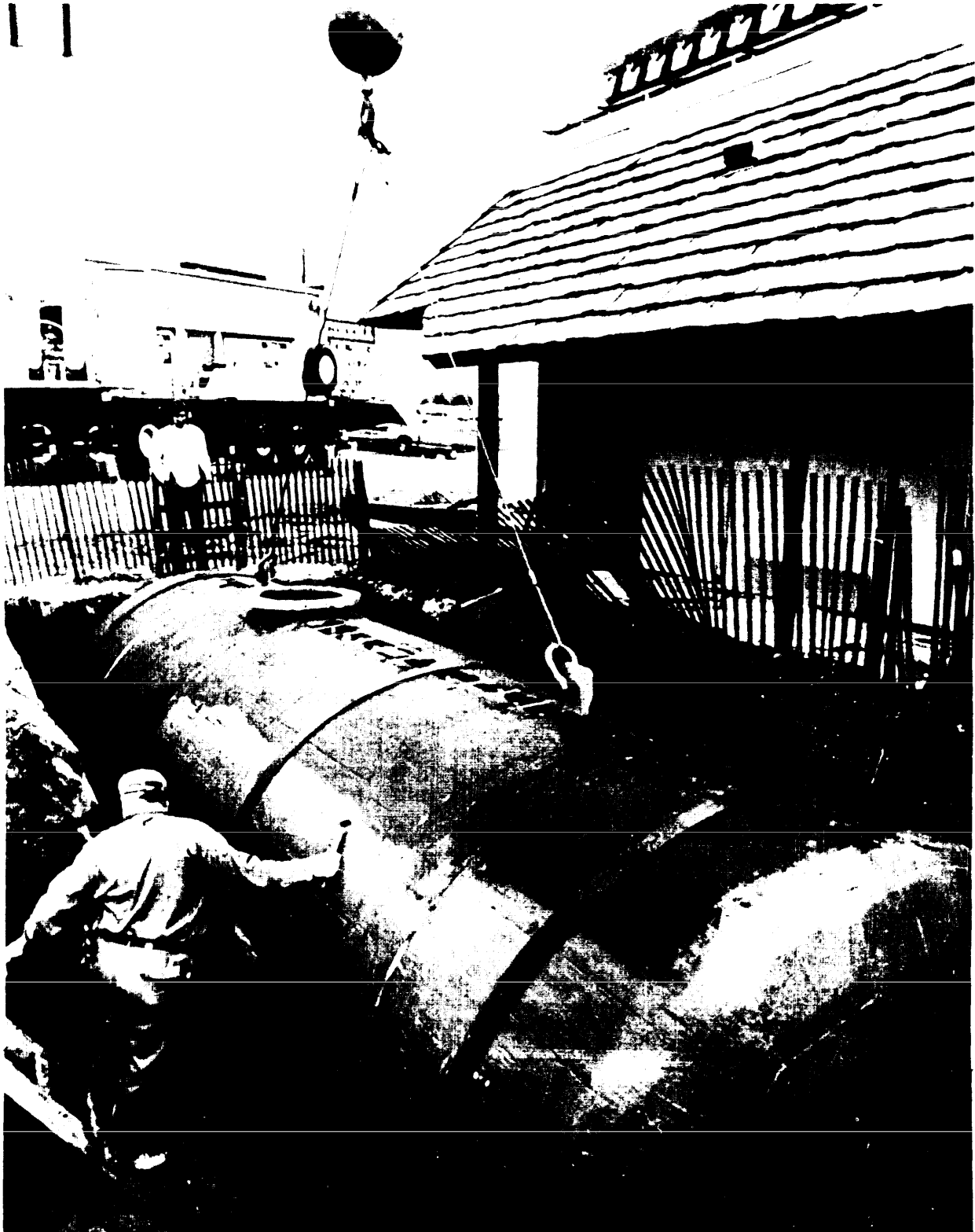
Figure XI-3.— Installation of Insulated, Underground, Storage Tank at Solar Heated and Air-Conditioned Burger King, Camden, N.J.
