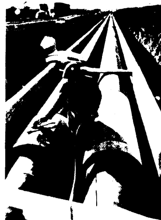
(2) Installation of district heating mains out to Kallerstad, a new industrial area
