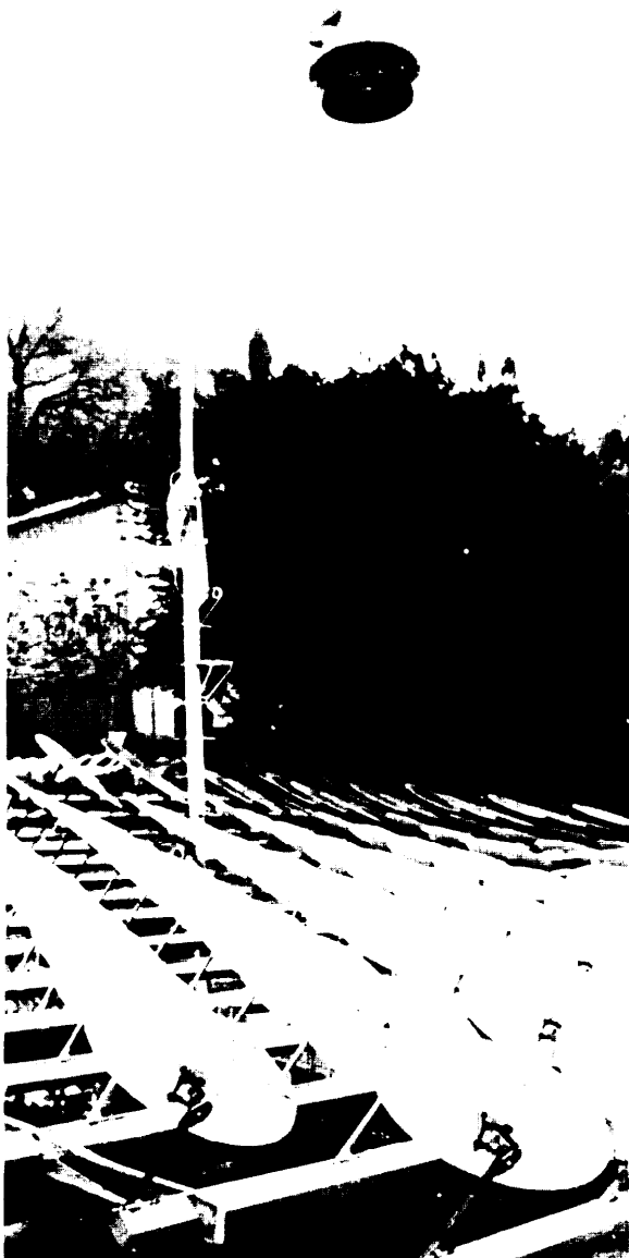
Figure VIII-27.—Francia 100 kW Solar Powerplant (Closeup of heliostats showing tracking linkage on back)
