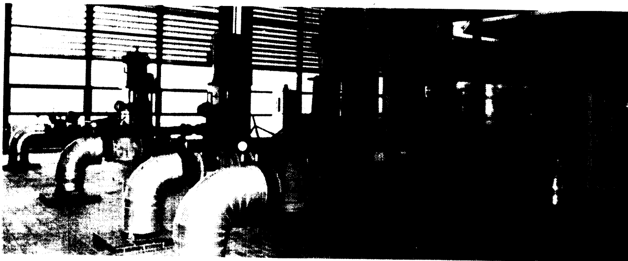
c) Main pumps in heating station
