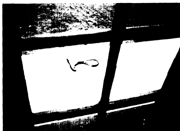
The imitation snake represents a “low-tech” solution to the problem of damage from bird droppings.
