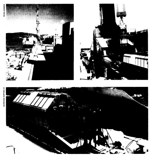
The Murmansk Shipping Company's Atomflot facility showing the dock and service ship Lotta where spent nuclear fuel is stored (top left); a railroad car used for transporting spent nuclear fuel from Atomflot to the reprocessing plant at Mayak (top right); the dockside crane transferring a spent tie/ shipping cask from (he service ship Lotta to the railroad car (bottom).
